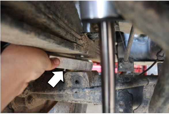
7. Safely lower the rear axle support and install the Eibach 1.0" lift block with the one pin facing the axle.
